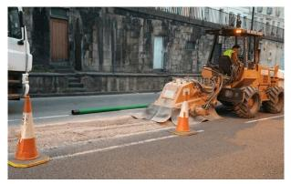
It is possible to cut one tram-track at a time for minimal traffic disrupting and no diversion of services. Photo: pipe-laying in Bath
