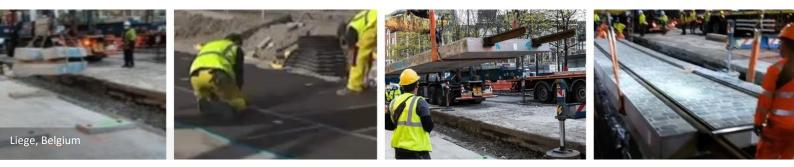
**Pre-formed track and pedestrian-friendly paving can simply be installed into a shallow trench on a "concrete float"** Example image shows rapid installation of prefabricated rail slabs with reclaimed cobble stones - placed evenly for comfortable walking. Optionally mounted on an elastic support to reduce noise and vibrations. Rails are welded together. Slabs fixed with fluid concrete. Suitable for rapid, night-time installation in areas accessible by large cranes.
