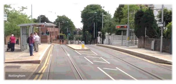
Fig. 21 - Example of a narrow road tram stop. All traffic share, cyclists routed behind tram shelter
